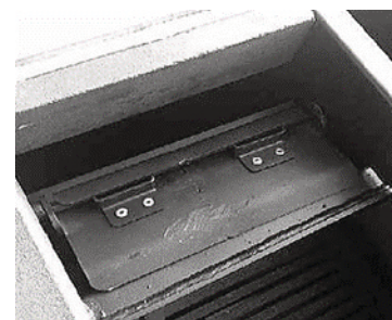
Open flue gas deflector (17) ⇒ Boiler efficiency significantly reduced!
