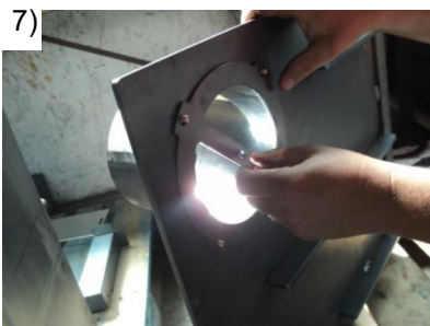
Afterwards, connect the chimney extension to the protective round cover and re-tighten the previous four bolts
