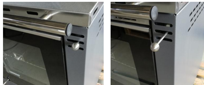
Closed flue gas deflector (17) Open flue gas deflector (17) ⇒ Boiler efficiency significantly reduced!
